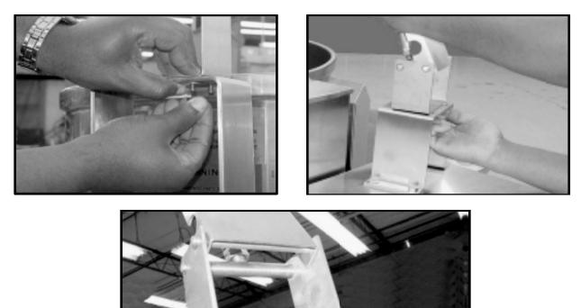
2.2 Assemble the actuator to the three studs on the domed cover and secure using thread locking compound and the dome nuts supplied in the cover kit. Tighten the dome nuts to 20 in/lb torque with a 1/4" open end or socket wrench.
